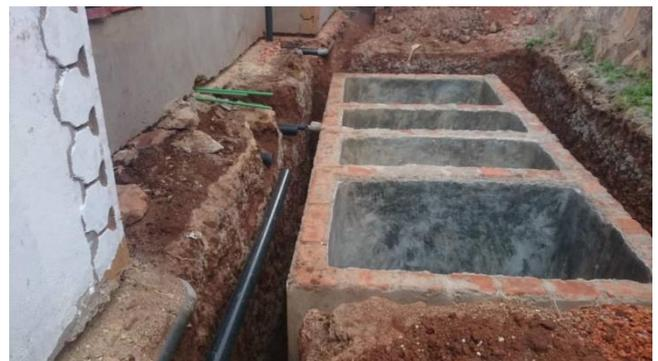
Gate hills Estate III will be using the individual septic tank which is still under construction. Despite valid criticisms concerning the low treatment performance of the septic tank, it is very important to note that septic tanks can operate effectively, if properly designed, operated and maintained, with regular and professional desludging, transport, treatment, reuse/recycle or disposal of the septic sludge.
