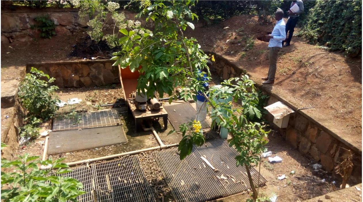
**Figure 28: Masaka Hill view estate sewage treatment system out of service**
