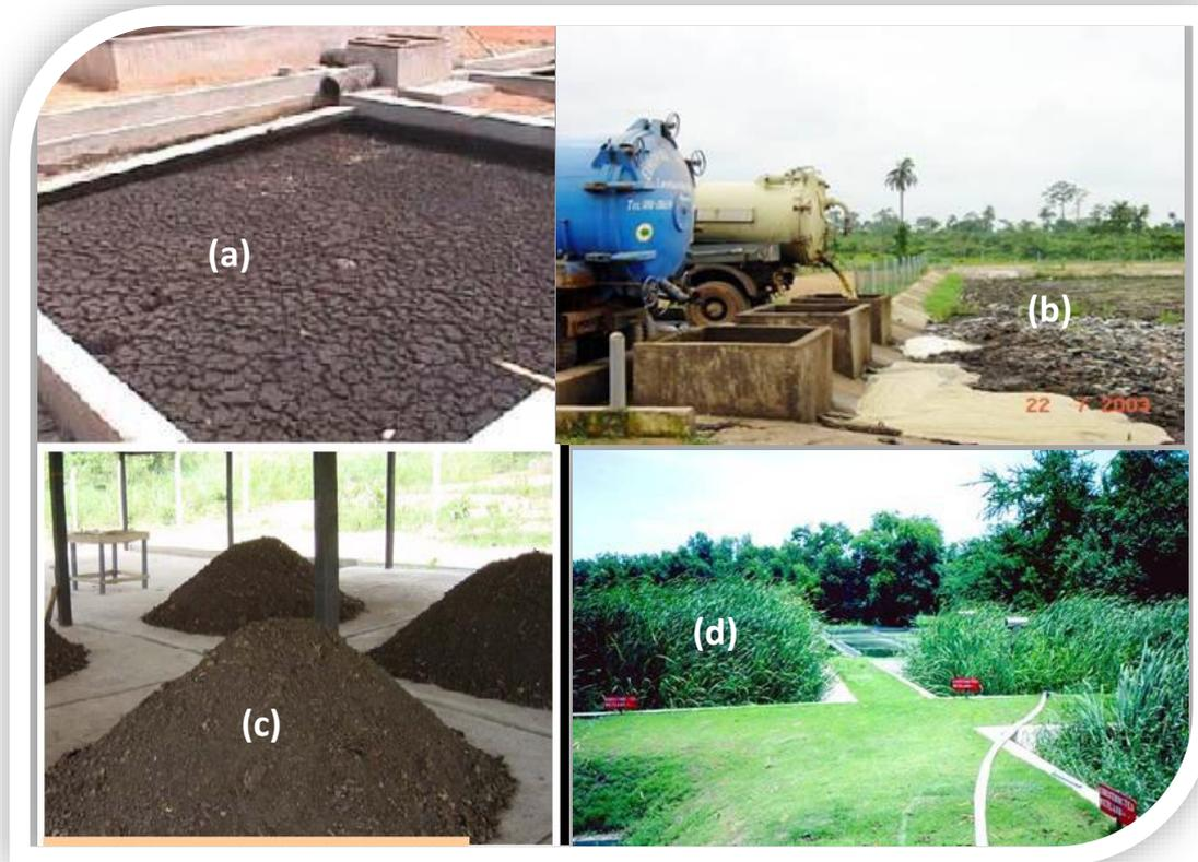
**Figure 19: Sludge treatment by drying beds (a), thickening (b), composting (c) and constructed wetlands (d)**
