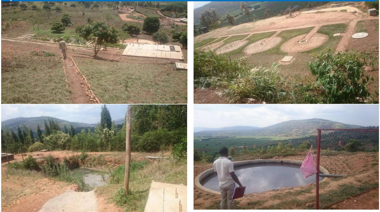
**Figure 35: Components of Mageragere sewage treatment system: Constructed wetland (a), Series of Biogaz Digester tank(b), effluent receiving pit before to be discharged into environment (c) and Influent receiving tank (d)**
