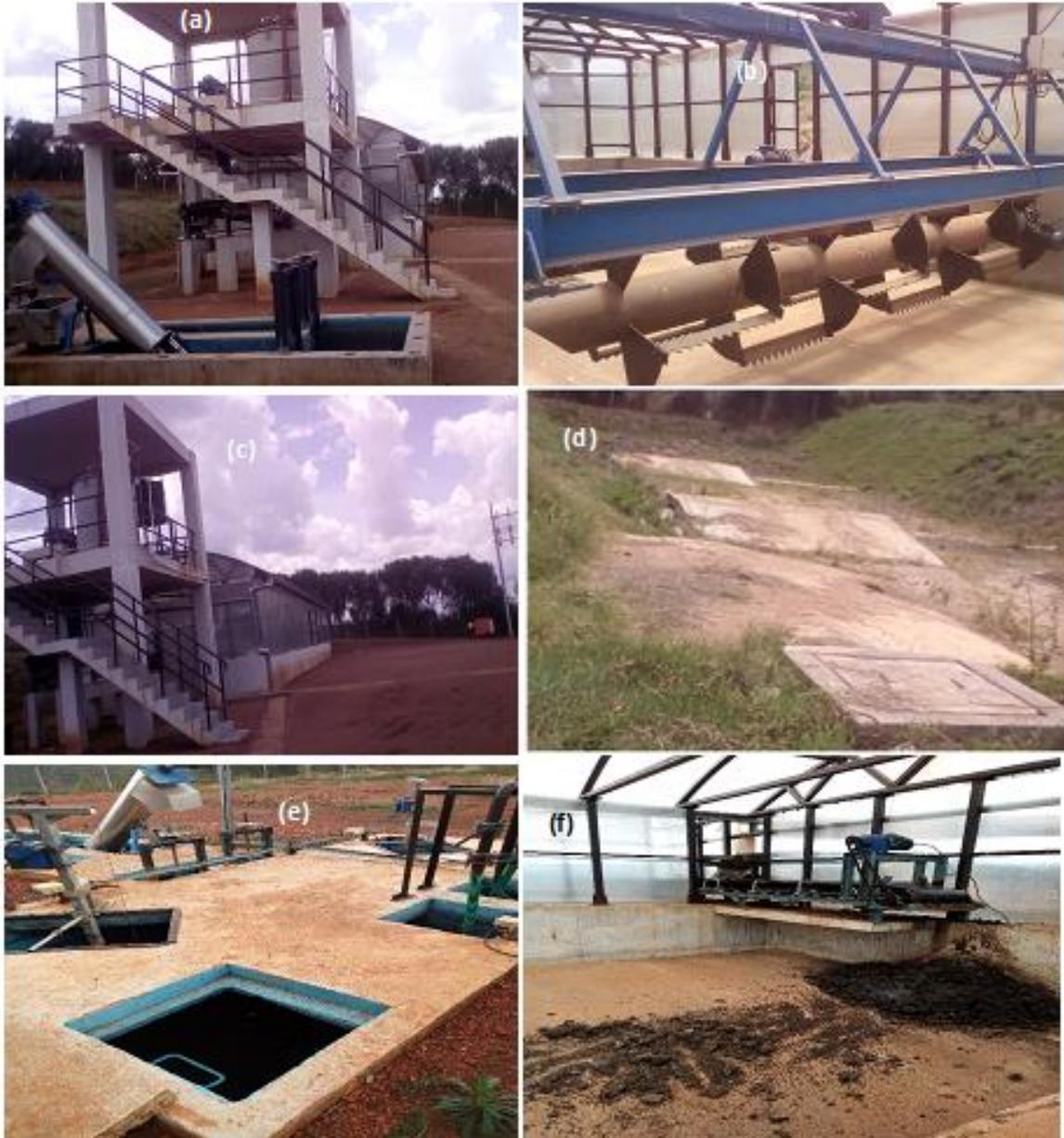
**Figure 46: Components of Faecal sludge treatment systems for Nyagatare, Kayonza, Nyanza and Gicumbi landfills including grit removal (a), Screw press for thickening sludge(b), Green house for solar drying bed (c), infiltration pit for wastewater (d), Waste water treatment chamber (e), Treated and stabilized Sludge (f).**
